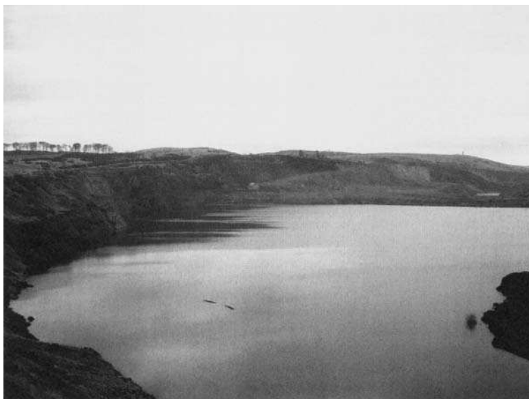
Fig. 1. (a) The main working pit (western basin) of the Westfield Opencast Coal Site, Fife, Scotland, as it appeared in the height of its productivity in 1974 (after Robins 1990). The far side of the pit is the highwall, 245 m in height, the outermost benches of which lie along the Ochil Fault, through which considerable quantities of groundwater entered the mine, as explained in the text. (Photograph: British Geological Survey, catalogue number D 1748, used with permission.) (b) The Westfield site viewed from approximately the same position on 12 December 2001, showing the pit lakes that have developed in the mine voids since coaling ceased. (Photograph: P Younger.)
